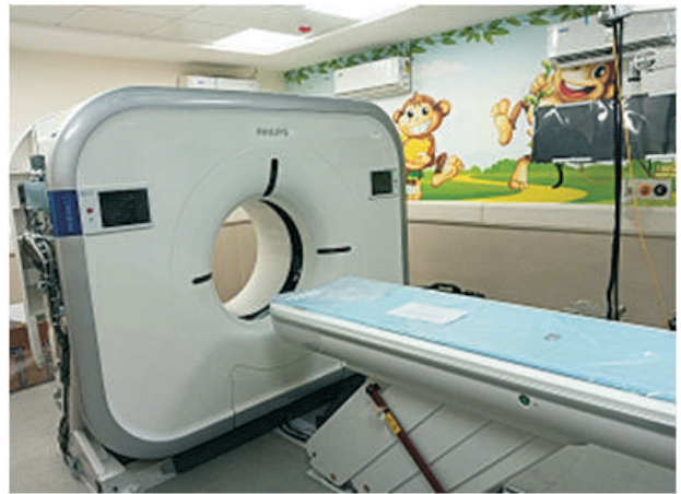
CT SCAN- 128 SLICE UNDER INSTALLATION
